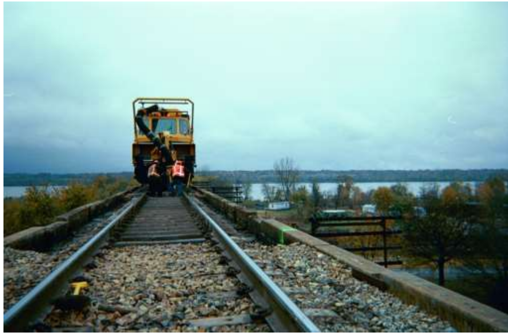
Undercutting Bridge Deck
