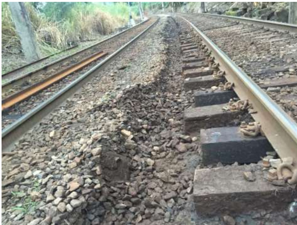
After Ballast Excavation - June 1, 2015
