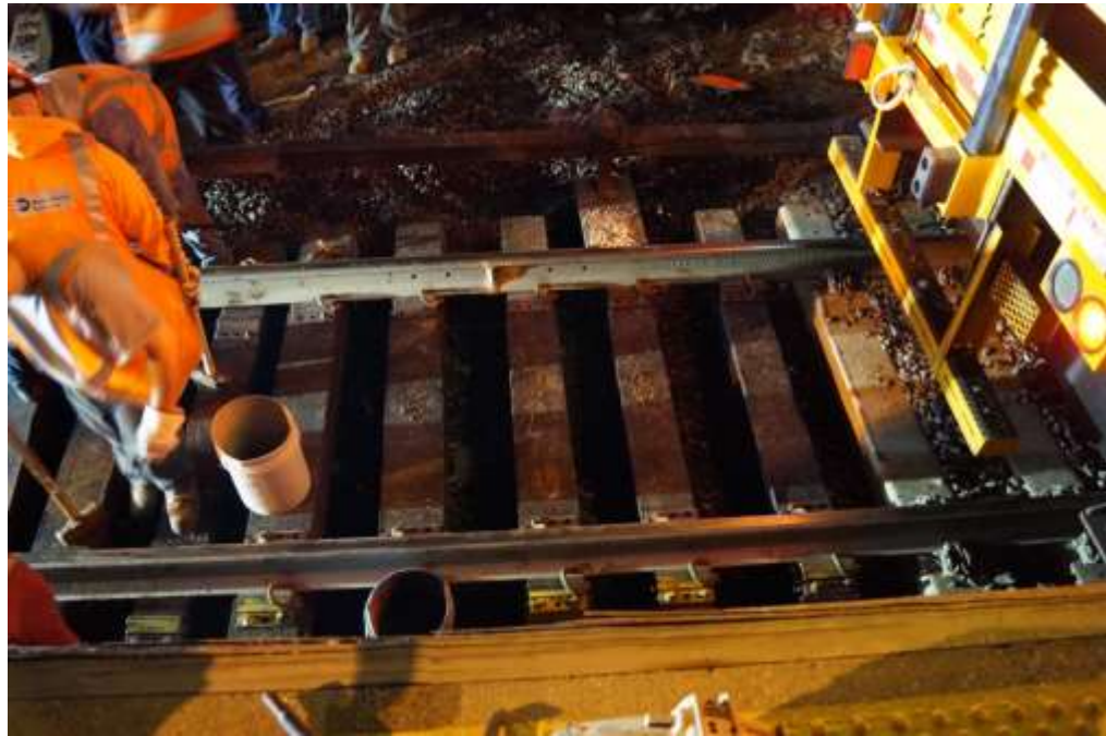
New Ties Being Secured to Rails and Reattaching Third Rail
