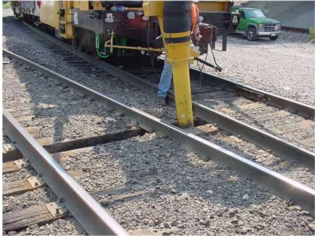
Undercutting Switch and Turnout
