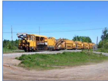
Pulling 4 Material Handling Cars
