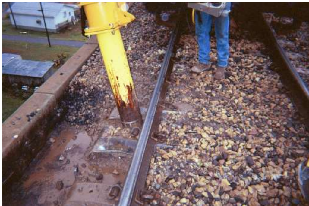
Bridge Deck Cleaning
