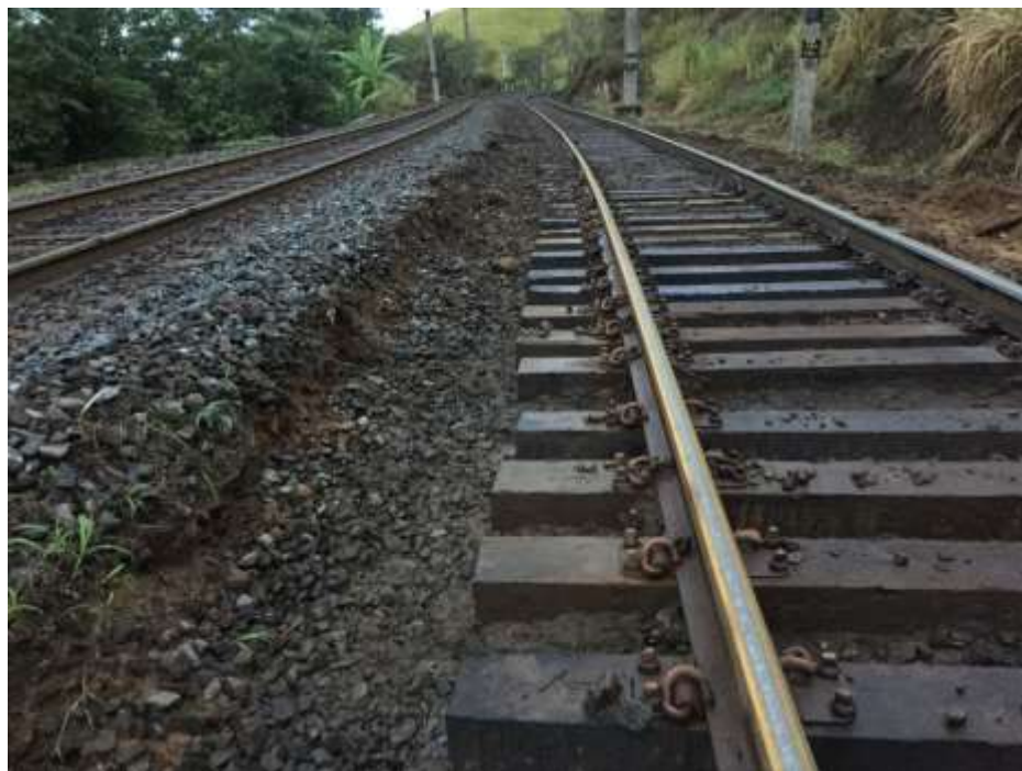
After Ballast Excavation – June 2, 2015
