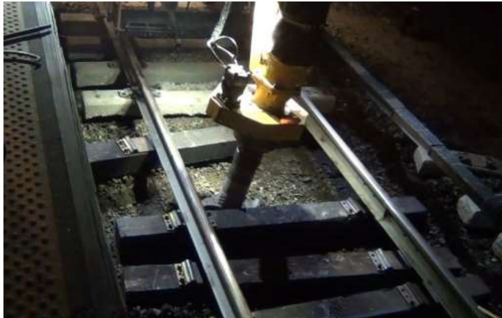
Railvac Staging New Ties Under Rails for Installation
