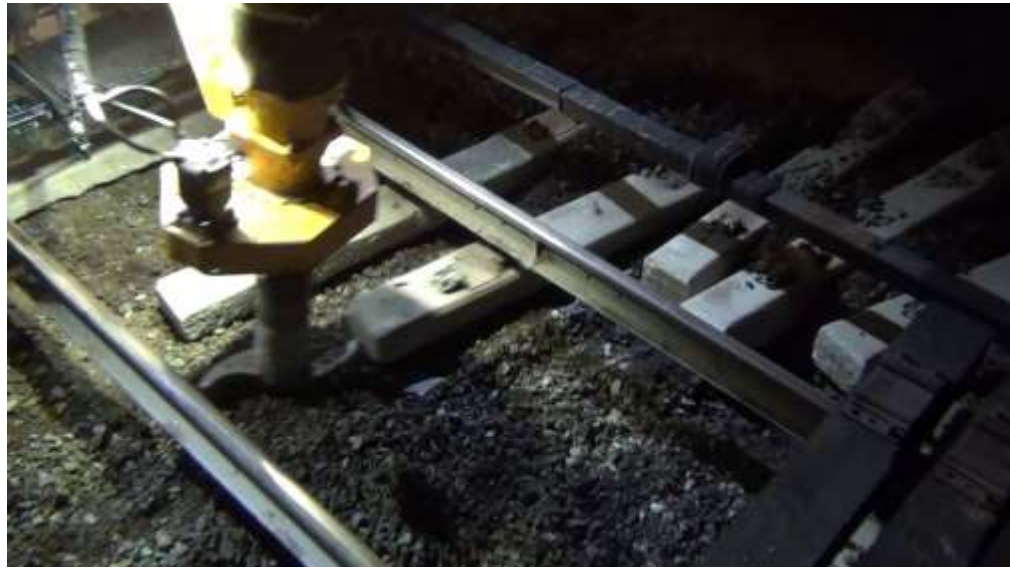
Railvac Sliding Dropped Ties onto Right-of-Way Under Third Rail
