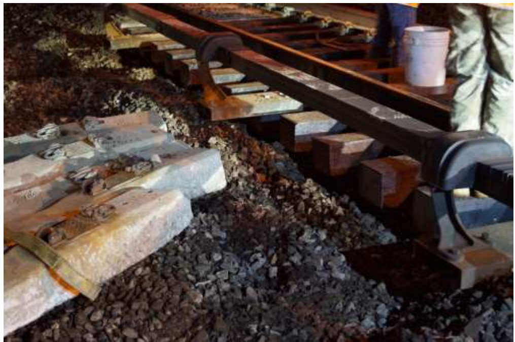
Track Waiting for Removal of Old Ties, New Ballast and Tamping
