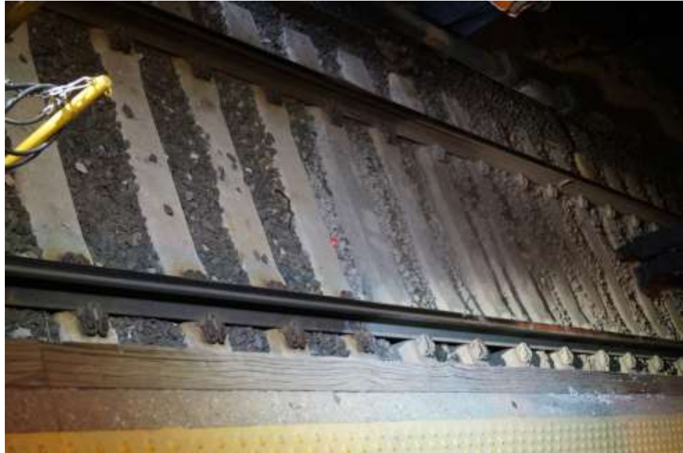
Condition Before Undercutting
