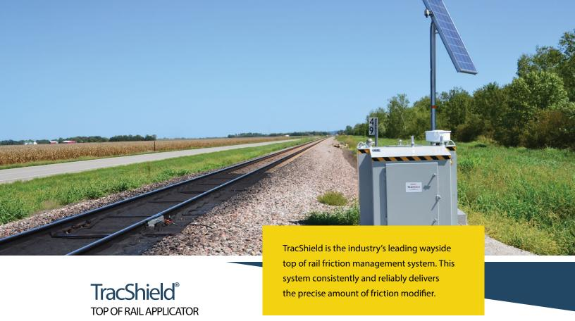
TracShield is an intelligent top of rail wayside friction management system. It senses the passing of train wheels over the TracShield's durable sensors and automatically dispenses a controlled amount of friction modifier to the top of the rail. Loram Technologies offers three different sized TracShields that provide options to select whether a smaller footprint, a large capacity tank, or a combination of those two is the most important feature.
